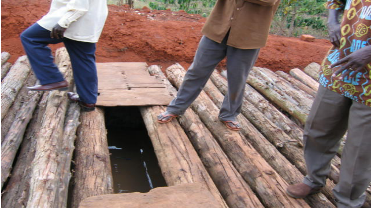
Construction of underground water reservoir
